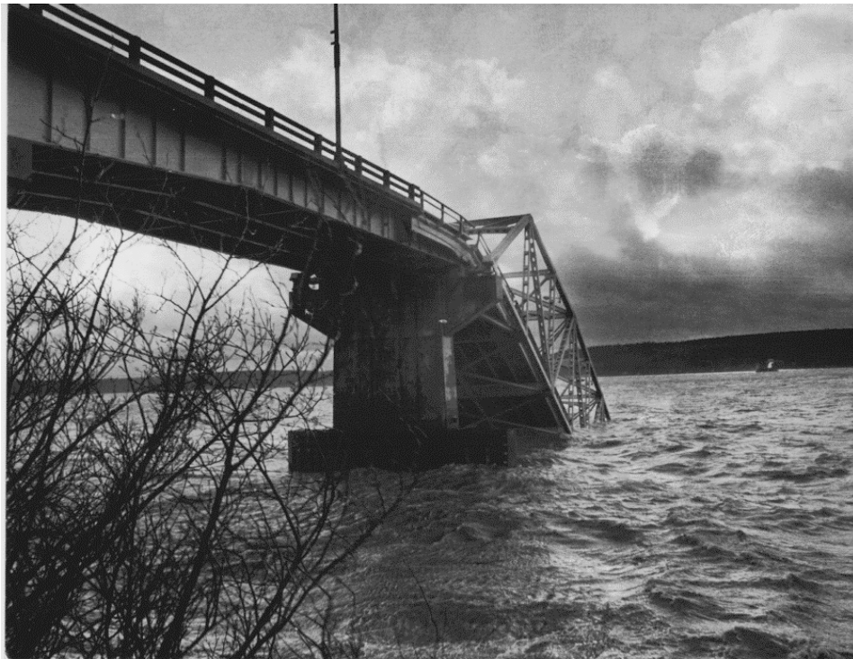
Winds of over 100 mph resulted in the failure of the western section of the Hood Canal Bridge on 13 February 1979.
