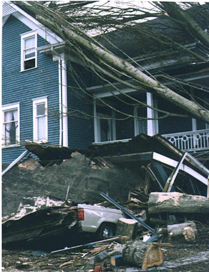
Most windstorm damage in the Northwest results from fallen trees, as illustrated by this photo of a home in north Seattle after the relatively weak windstorm of 30 March 1997
